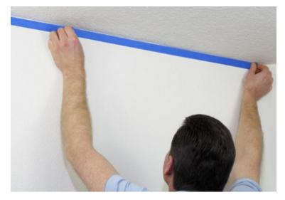
Figure B.1: Masking Procedure [33]
